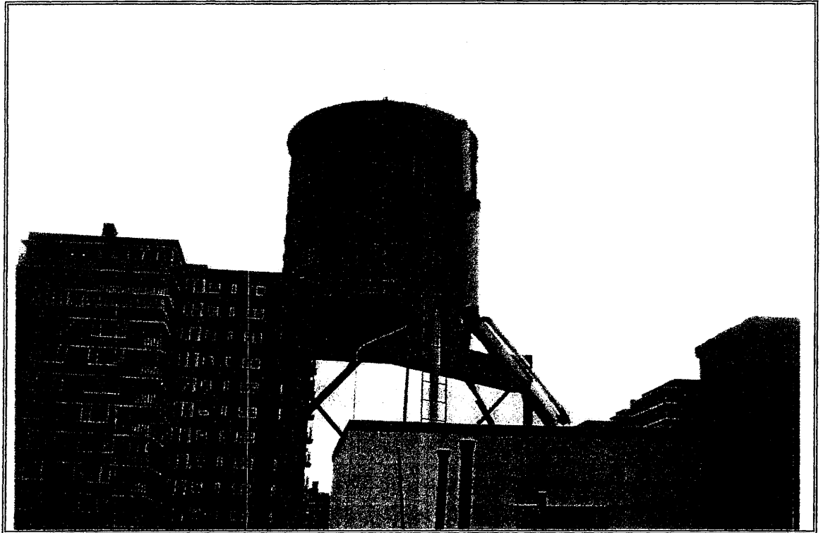
View of the water tank
